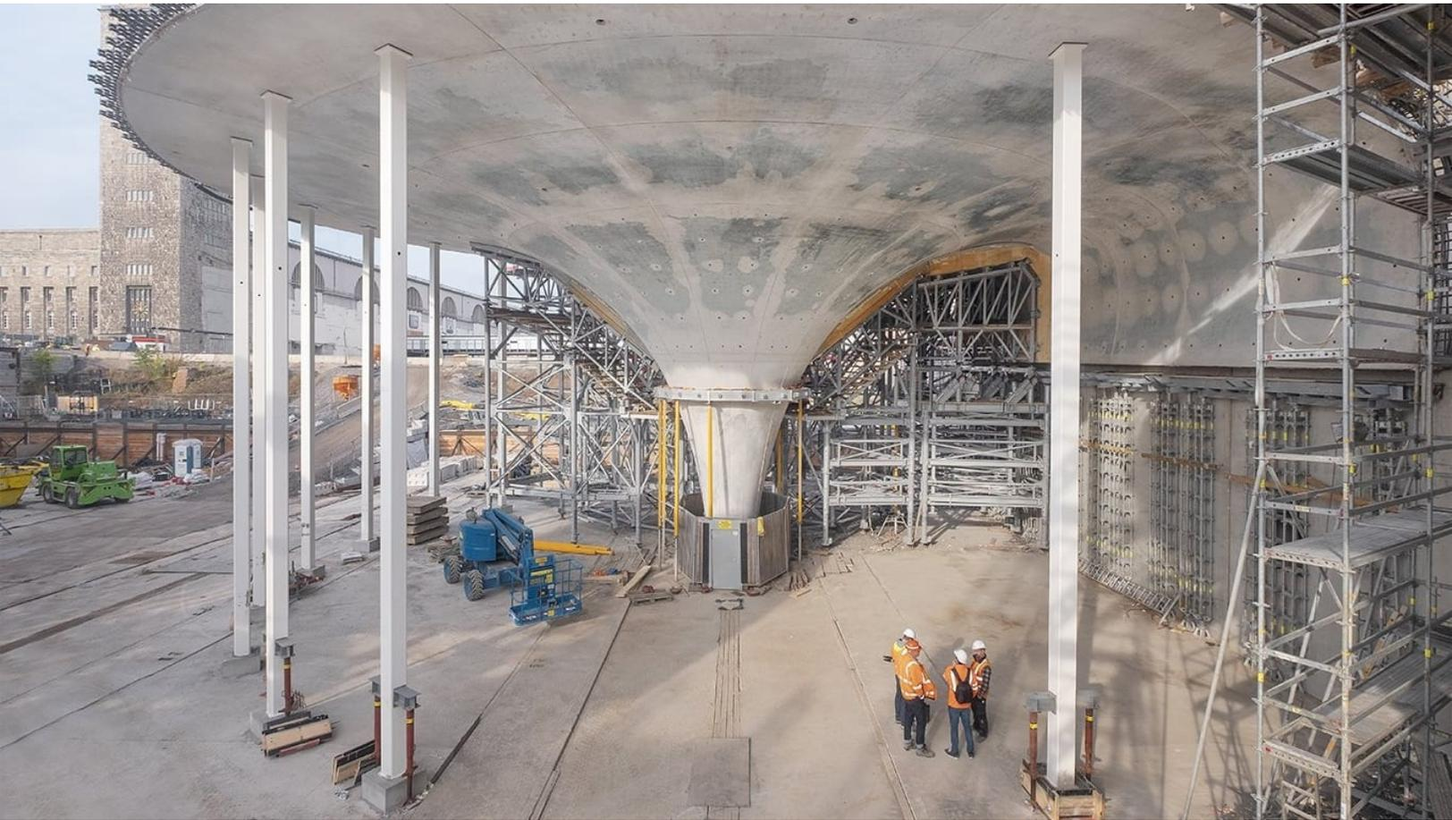
The first of 28 chalice-shaped columns that will combine to hold the roof of Stuttgart's new underground through station was completed in October 2018. copyright: Achim Birnbaum
