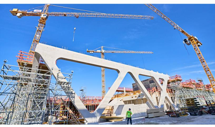
ZÜBLIN's Bavaria Subdivision produced the complex structure using in-situ concrete. (Copyright: Ed. Züblin AG/Photographer: Gert Krautbauer)
