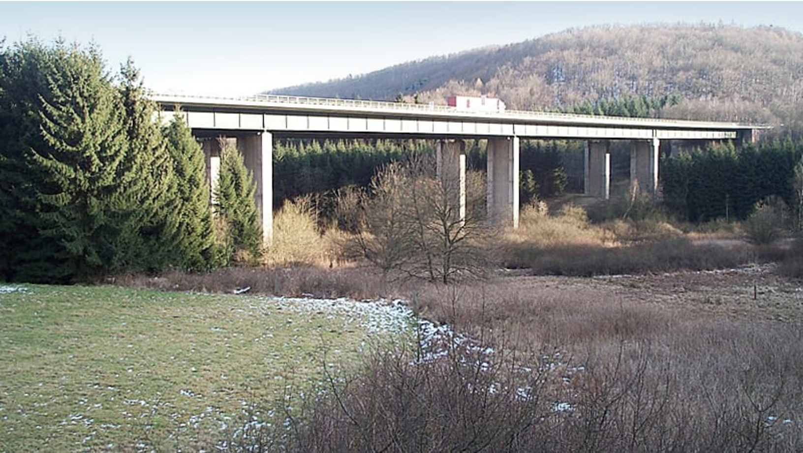
The Grumbach Bridge along the A6 motorway before its renewal.
